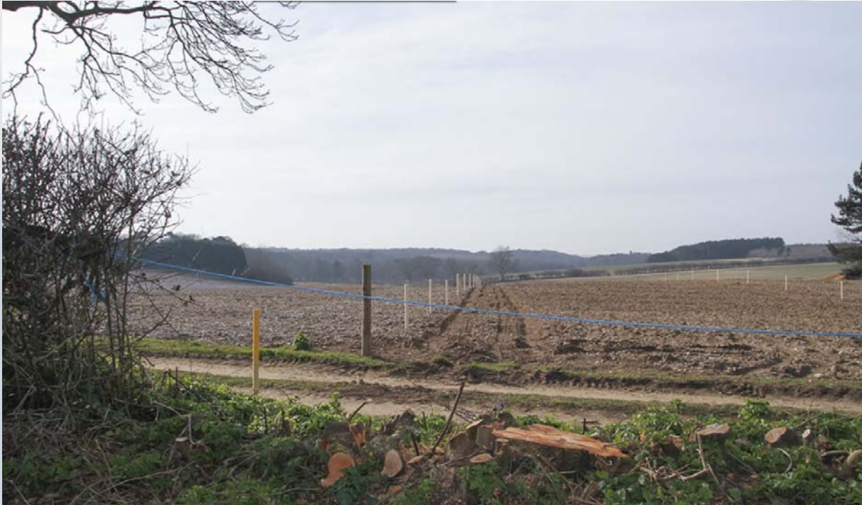
Hedging and Fencing on Dudgeon 132kV Onshore Cable Route
